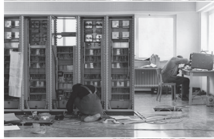
1968 Interior construction of the operating room
