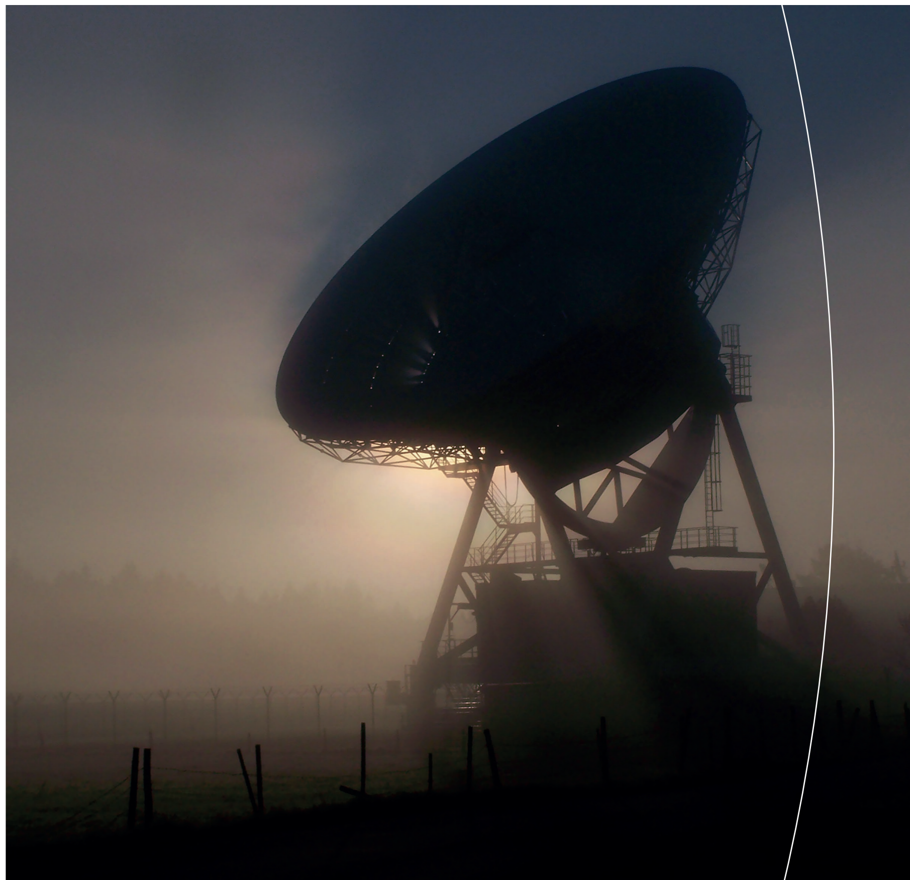
The landmark of the Weilheim ground station: the 30-metre antenna. It was built to send commands to the HELIOS 1 and 2 spacecraft, which were launched in 1974 and 1976 respectively.
