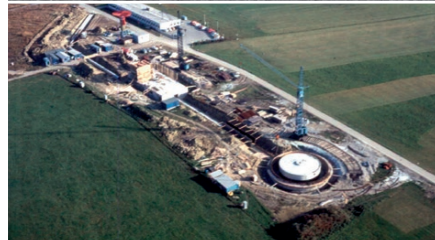
1972 Construction work on the HELIOS command station
