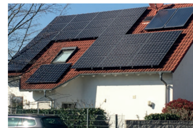
For the automated detection of solar power systems, the software must be able to distinguish between different elements in order to avoid misclassifications. Roofs like this are used for test purposes; here, both solar-thermal and photovoltaic elements can be seen, but also a roof window, which must not be incorrectly labelled as a solar power system.
