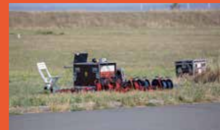
Measurement data logging unit and cable drums
