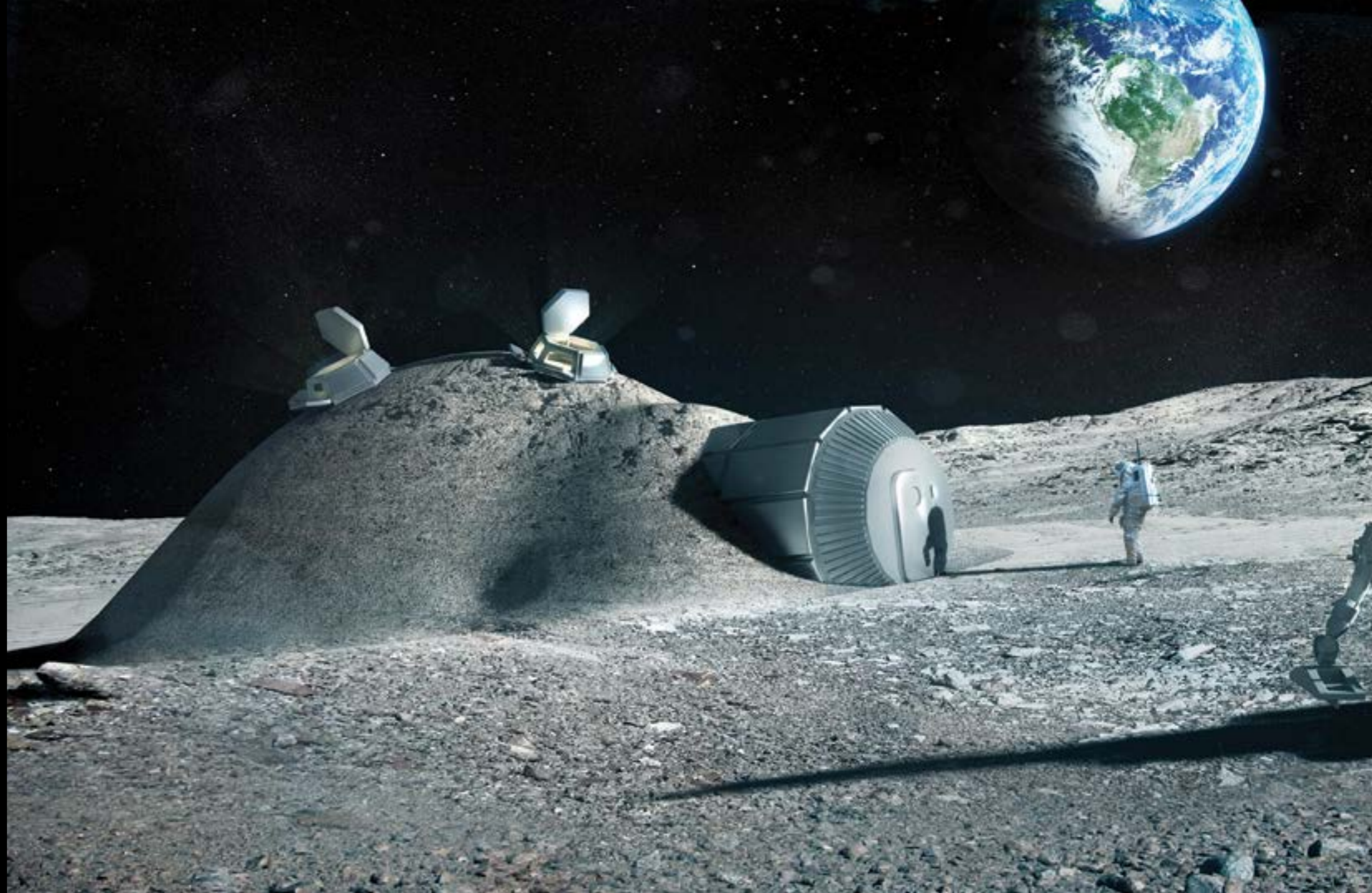
Artist's impression of a 3D printed lunar base made from layered regolith (ESA/Foster + Partners)
