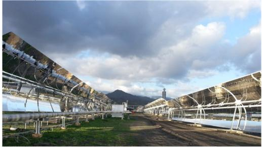
In the DUKE (Durchlaufkonzept – Entwicklung und Erprobung [Cycle Concept – Development and Testing]) test system, the steam needed to generate electricity is produced directly in the receiver tubes of the parabolic troughs. Intermediate steps employing a heat transfer medium are no longer needed and higher operating temperatures are possible.
