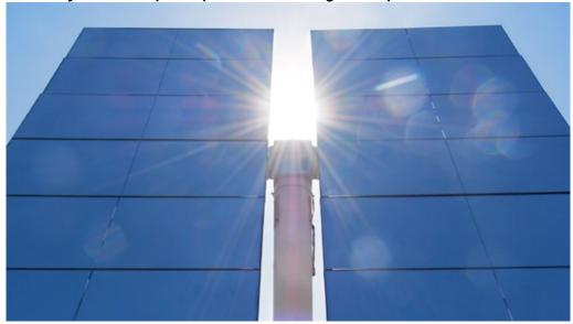
The Sun behind the heliostat of a tower power plant. When operating the power plant, the mirrors on many heliostats direct sunlight to the tip of a tower where temperatures of up to 1000 degrees Celsius are generated. Electricity is produced via a turbine and a generator. Tower power plants operate at higher temperatures, which helps to make electricity generation more efficient.
