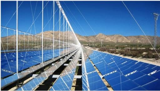
Fresnel collectors consist of numerous slightly curved mirrors, which focus solar radiation onto a central absorber pipe. In this pipe, water can be evaporated and superheated and the thermal energy is then converted into electricity by a steam turbine. The Puerto Errado Fresnel collector solar thermal power plant is located in Murcia, southern Spain.
