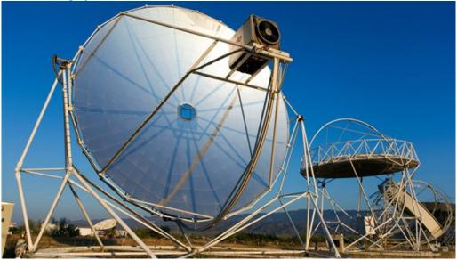
In Dish-Stirling systems, a parabolic mirror concentrates solar radiation into a focal point, where the Stirling motor is placed. Heat energy is transformed into mechanical energy by the Stirling motor. As a general rule, a generator then uses the mechanical energy to generate electricity.
