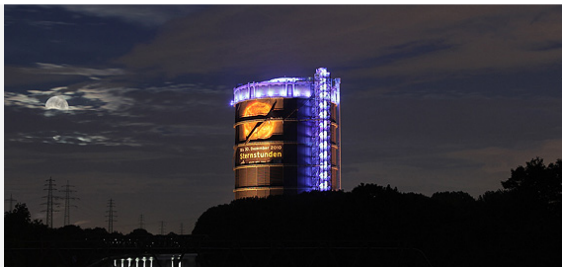
'Out of this World' in the Oberhausen Gasometer
