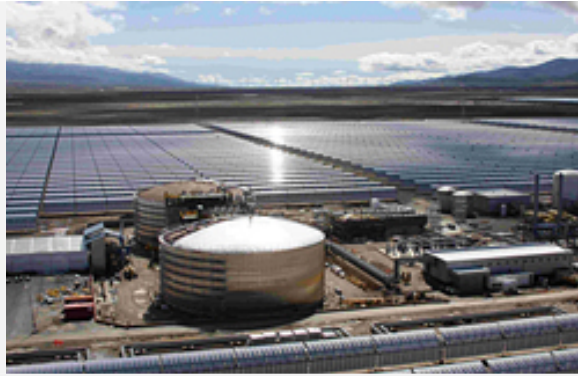
Andasol 1: The world's largest solar power plant delivers power to 200 000 people
