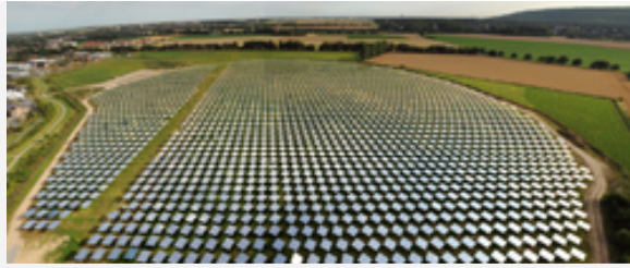
Heliostat field: over 2,000 movable mirrors
