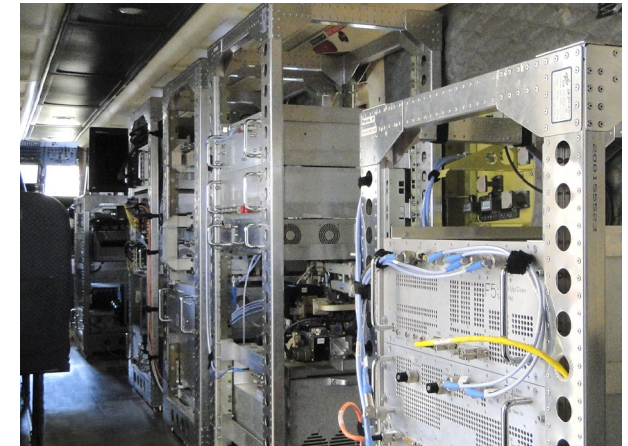
The F-SAR instrument installed in the cabin of the Do 228 aircraft. Standard instrumentation racks hold the radar's electronics units.
