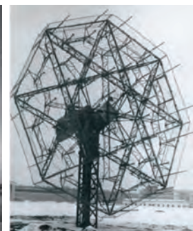
Experimental set-up of an electronic switched direction finder (left), VHF monopulse tracking antenna for satellite signal reception, diameter 11 m (right).
